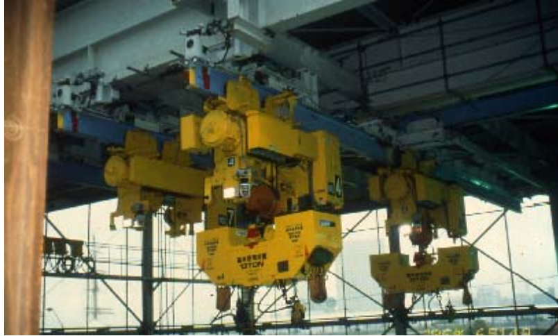
Figure 15*: Automated construction site SMART(Shimizu) seen from above Figure 16*: Two of 22 robotic trolleys for transporting and positioning of beams, columns, floor panels, building services units and facades
