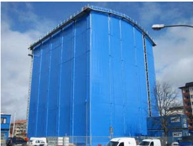
Figure 20: On site factory of NCC Komplet [4].
