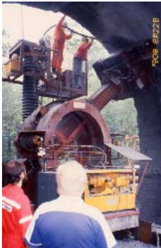
Figure 9*: Robotic concrete roller for tunnel construction Figure 10*: Robotic tunnel segment assembly unit
