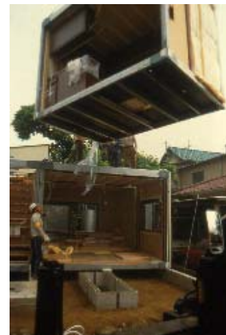
Figure 7*: Quality End Control of a box unit with bathroom from a flexible manufacturing system Figure 8*: Onsite assembly of a box unit house
